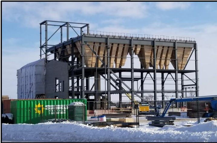
New mill with hoppers installed with North wall in place.
