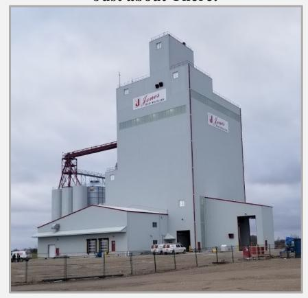
The new George Robert Jones Bulk Production Plant is nearing completion. In mid-November the boilers were fired up and tested. Currently the technology components of the mill are being installed; while wiring and other utilities are nearing completion. This month we will see some of the first tests of the mill itself. At this point we are on schedule and feel the first feed will be shipped sometime in January. Stay tuned for more updates!
