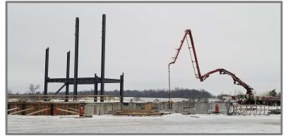
The new **George Robert Jones Product Plant** is beginning to show life above ground. Much of the basement - which houses some of the mixers and the boiler room is complete. The frame for the building portion of the mill is currently being installed. JFM salutes the many contractors that have been working on this project and thank them for their tireless efforts through a tough grind of fall weather.
