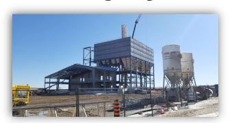
Despite a difficult winter for weather, the new George Jones Bulk Production Plant remains on schedule. Above you can see the framework for the utility and control rooms out front as well as the bin housing in the background which is roughly 50% complete.
